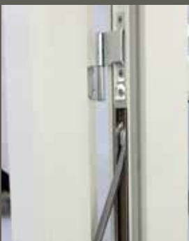
Hidden wiring between the frame and the lock, positioned within the frame.
